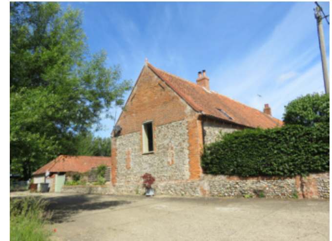
South elevation showing glazed door opening of Lantern Barn at the north end of Lower Hall Lane
