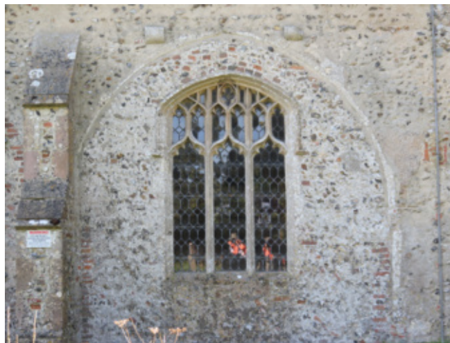
Window on the north elevation of All Saints church
