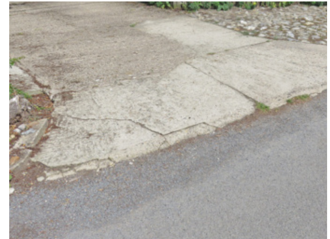
Large concrete splay
