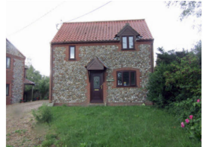
Modern house located on The Street
