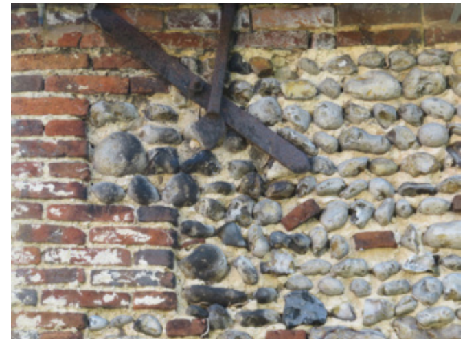
Regular overflowing of water from missing, damaged or inadequately sized rainwater goods causes damage to the historic fabric
