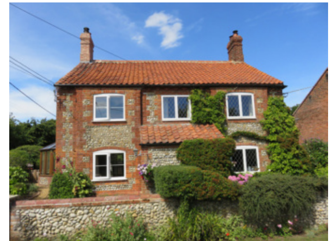
Front elevation of 22-23 Bale Road
