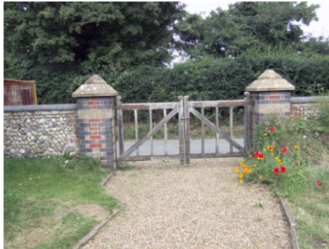
Cobble flint and red brick wall around the churchyard with attractive gate piers and timber gate
