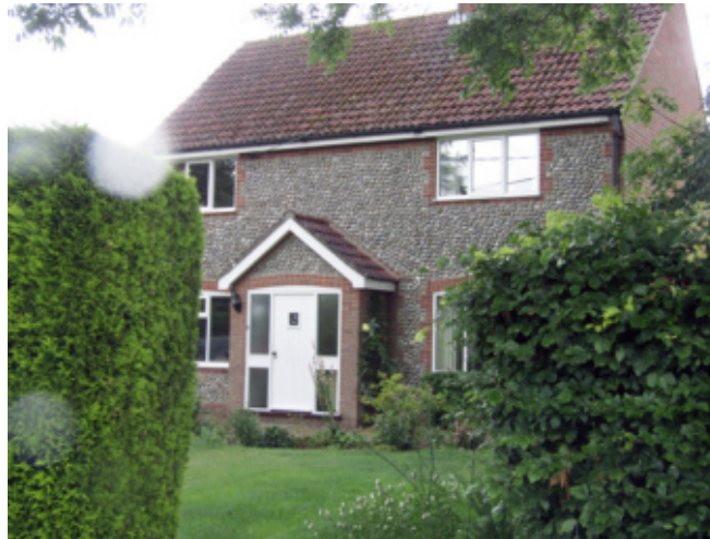
Modern house located on The Street
