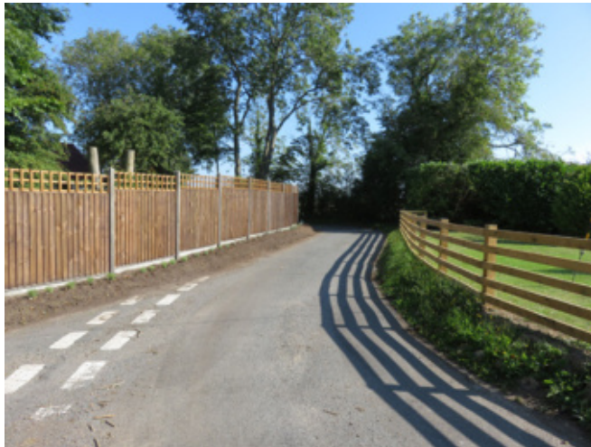
Timber fences on the boundaries of houses north-east of The Street. Fencing, especially close boarded fencing with trellis between concrete posts is not in keeping with the character of the Conservation Area
