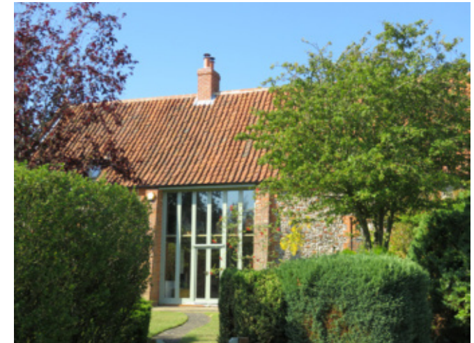
East elevation of Sharrington Hayloft converted barn showing glazing in barn door opening
