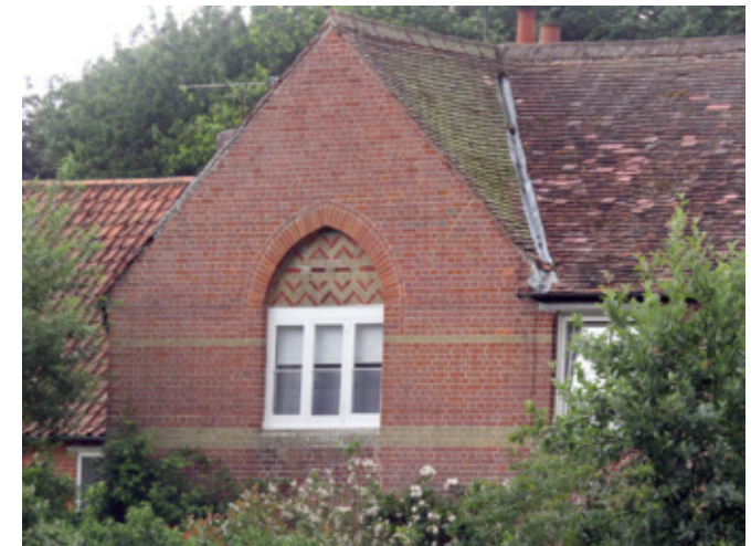
Detail of window on The Old Rectory
