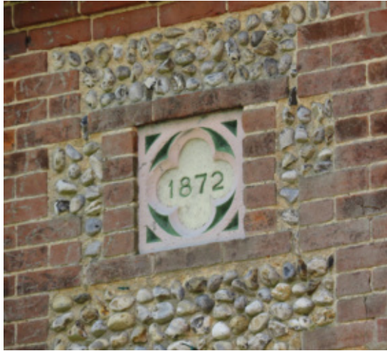
Date stone in quatrefoil surround in terracotta
