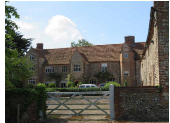
Front elevation of Sharrington Hall
