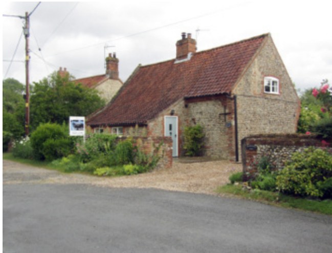
Medium sized historic house located on The Street
