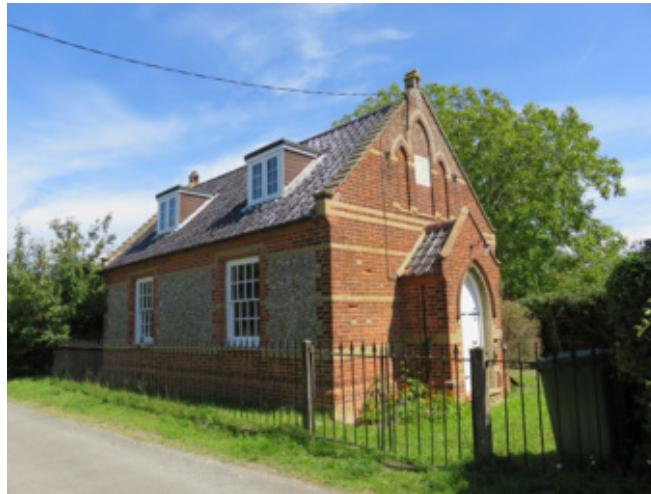
North and west elevation of converted Wesleyan Chapel
