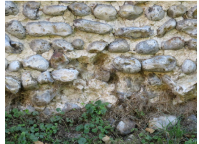
Eroded pointing causes loss of flints
