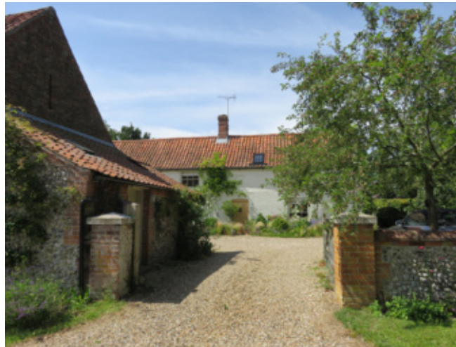
Front elevation of Daubeney Hall Farmhouse on Lower Hall Lane
