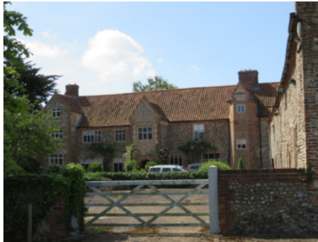
Front elevation of Sharrington Hall
