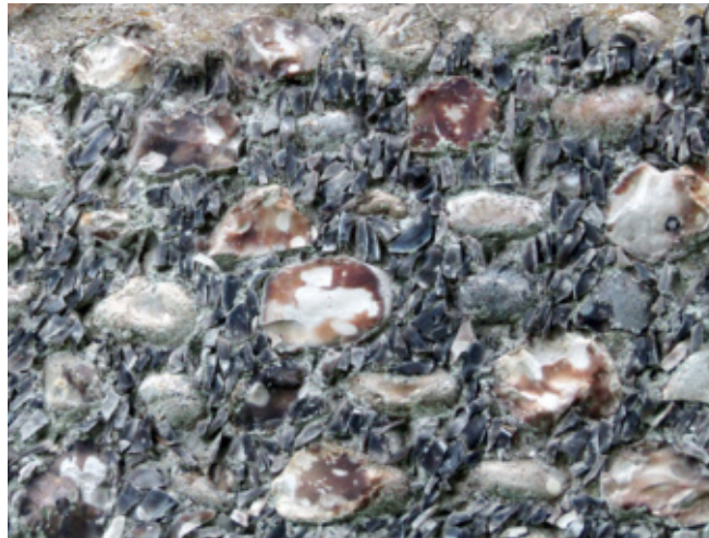
Flint galletting on Sharrington Hall Barn
