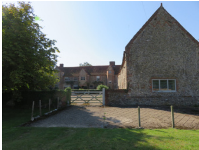
North elevation of Sharrington Hall Barn
